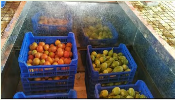
Zero Energy Vegetable Cooling Chamber in Umred Taluka, Nagpur (Source: RuKart)
